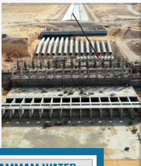
HAMMAM WATER TRANSFER PROJECT
